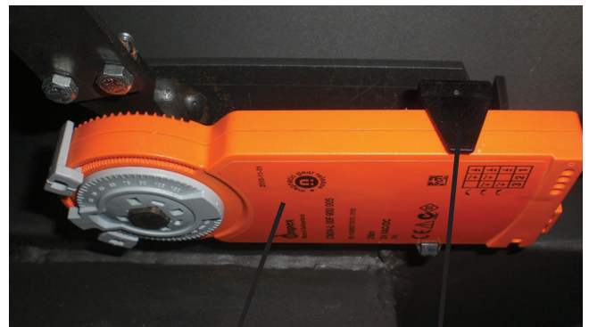
Servo motor Motor retaining clip
